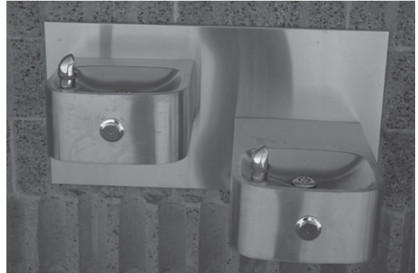
Fountains Connected to a Central Chiller
